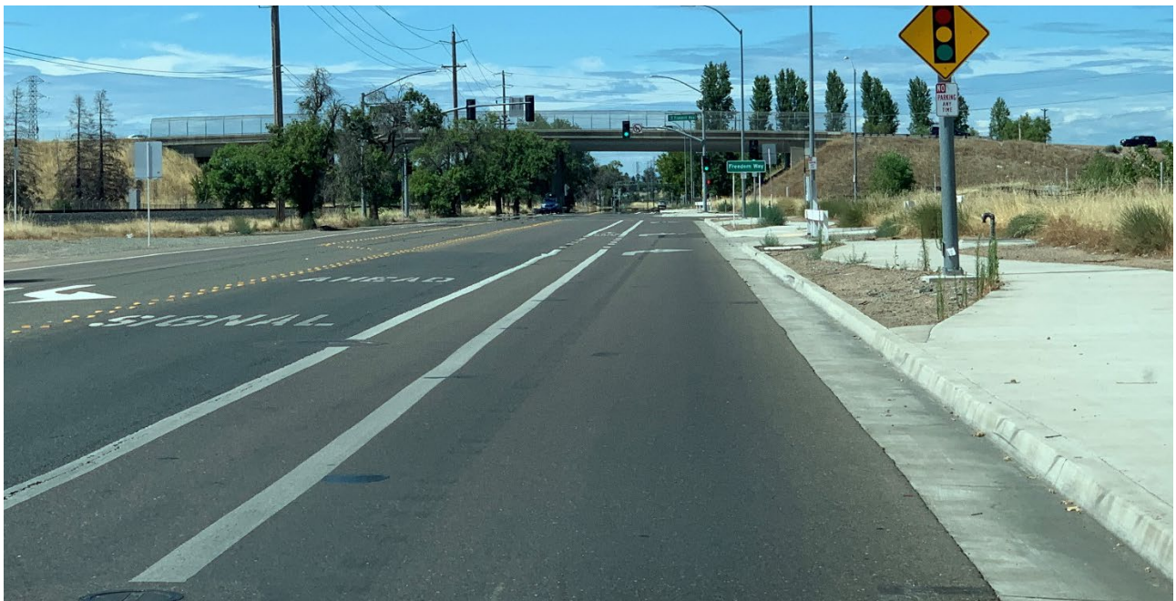
Image 5: View looking northbound on Industrial Avenue toward Driveway 2
