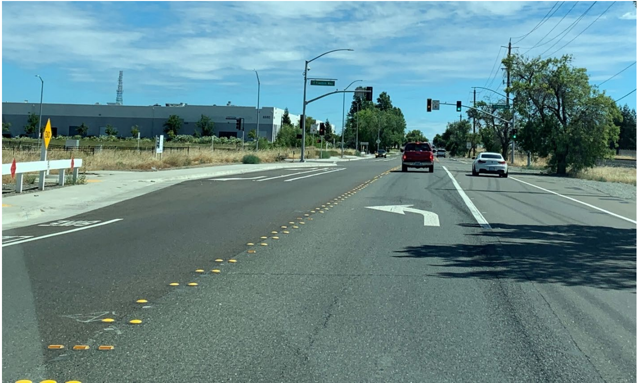
Image 4: View looking southbound on Industrial Avenue at Driveway 1 entrance
