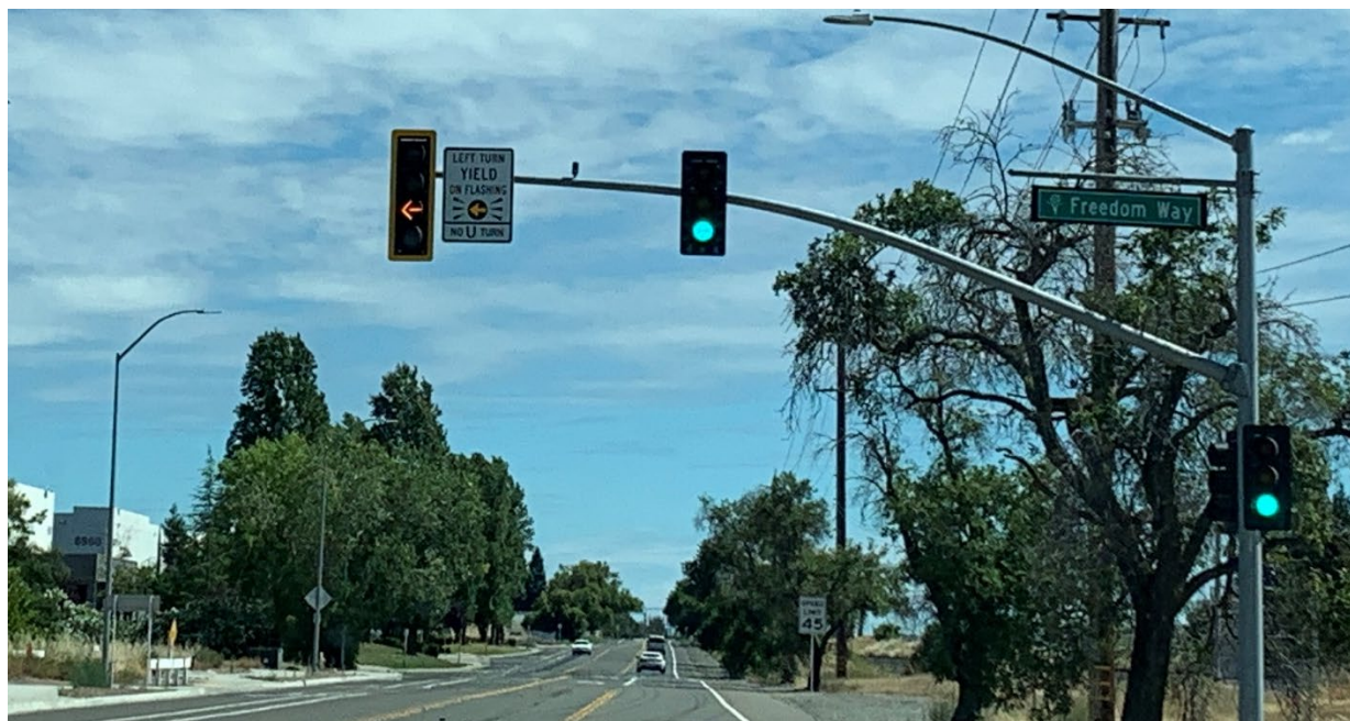
Image 1: Flashing yellow arrow for southbound left-turn lane on Industrial Avenue
